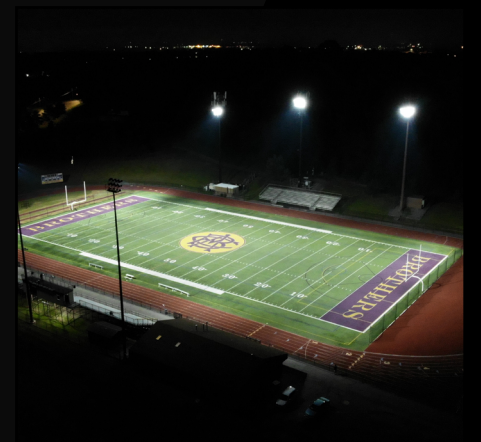
CURRENT SYSTEM AT NIGHT
