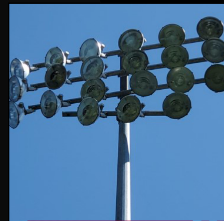
CROSS ARM CONFIGURATIONS
